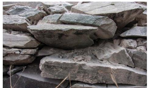
Fig. 5. Bulging plinth with eroded mud mortar (North-east).
