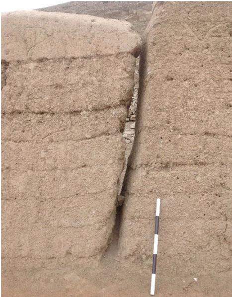
Fig. 2. Mud layers in a wall, it can see the concavity formed. Palace of Oquendo – Lima (Source: Torres, 2021).
