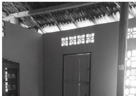
Fig. 3. Roof expansion over the wall, space for exit of hot air. (Source: Authors, 2021)
