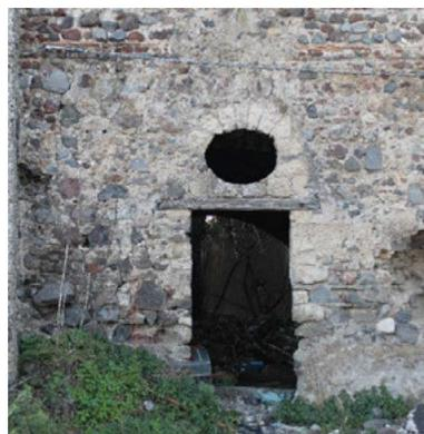
Fig. 5. Fortified house Fasano, detail of the access to ground floor: note the masonry construction 'a cantieri' and the flat-tenting surface of the masonry section using brick elements (Source: Ragosta, 2022).
