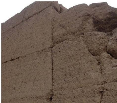
Fig. 7. Joint between modelled earth blocks. Huaca Tres Palos – Lima (Source: Torres, 2021).
