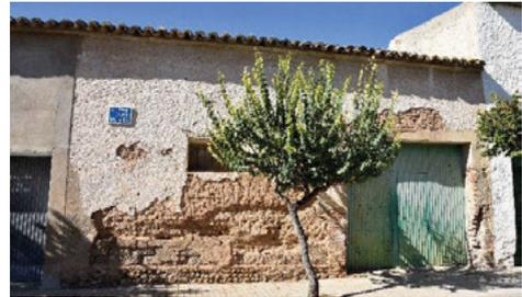
Fig. 6. Vernacular adobe building with visible erosion.
