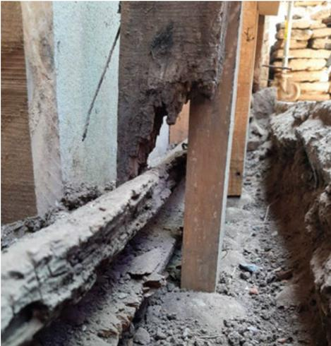
Fig. 7.a. Stone foundations and damage in bearing wooden elements in original walls (Source: Authors, 2021).
