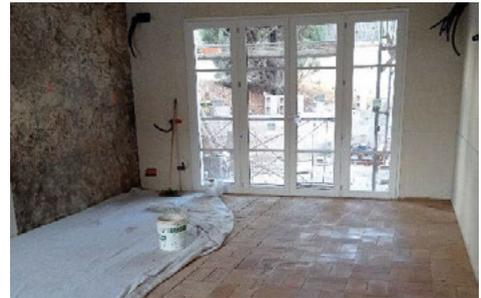
Fig. 10. Clay tiles already placed in living room, waiting for minimum 25 days complete drying (Source: Li Puma, 2021)
