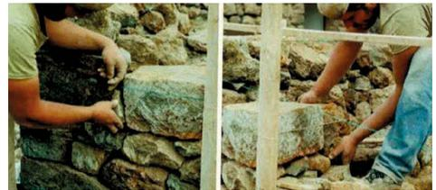
Fig. 5. Wooden scaffolding and line for the construction of a dry stone wall (Source: Progetto Medstone, 2002)
