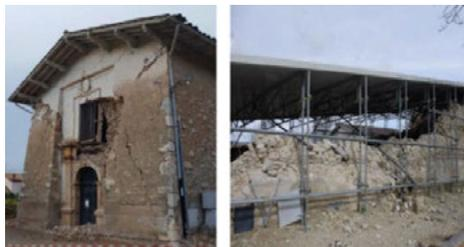
Fig. 3. The church of *S. Antonio Abate* after the earthquake of 24<sup>th</sup> August 2016 (left) and in 2017, after its collapse (right) (Source: <https://frascadorinorcia-noprofit.webnode.it/galleria-immagini/> (a); <https://www.iluoghidelsilenzio.it/frascaro-norcia-pg/> (b)).
