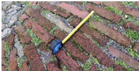
Fig.9. Old bricks with a rough appearance, with a slight tendency to disintegrate (Source: Fratini).
