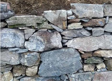
Fig. 1. An authentic stone-dry walls made using the Moltrasio limestone (Photographed by the author, January 2022)
