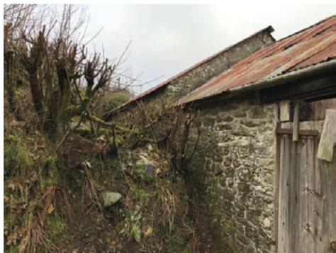
Fig. 7. Build-up of spoil and tree growth against south wall prior to excavation (Source: Jonathan Rhind Architects, 2019).
