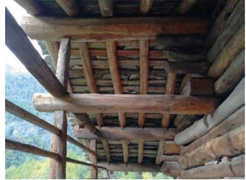
Fig. 5. Detail of the structure of the roof built with three frames, carrying stone labs (Source: Di Paola).
