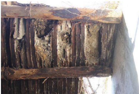
Fig. 9. Fortified house Casillo. Wooden ceiling with chestnut beams and second-arybeams ('chiancarelle') and flooring stratigraphy (Source: Ragosta, 2022).
