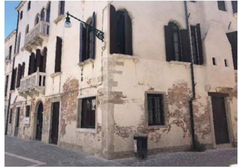
Fig. 5. New thick plasters cannot withstand the effect of rising damp for long in Venice: the above example is less than a decade old (Source: Squassina, 2021)
