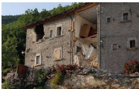
Fig. 2. Overturning of façade in a clogging unit (Noeria)
