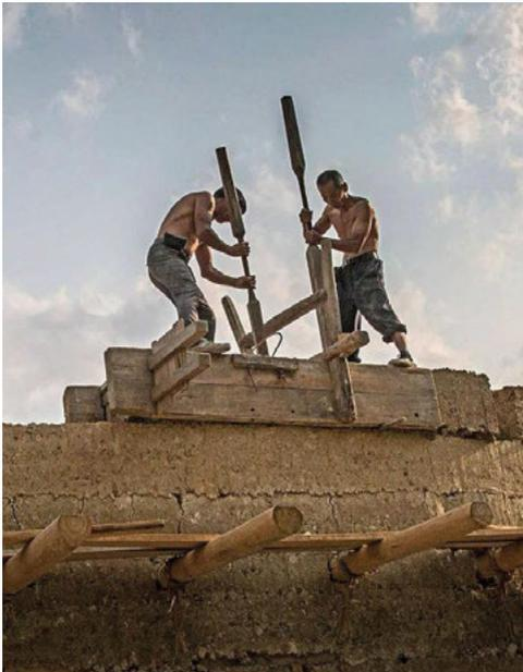
Fig.12 The formwork used in Tulous (Source: Chen, 2016, [www.163.com/dy/article/E9GLU3K10521AJ1J.html](http://www.163.com/dy/article/E9GLU3K10521AJ1J.html))
