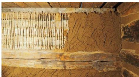
Fig. 4. House No. 14 and mud plaster application on reed mesh, the plaster is coarsened for easy topping coat adhesion as well as prevention of shrinkage cracks, Lhota Rural Reservation, Česká Lípa District, Liberec Region © Martin Cernansky, 2020, NHI
