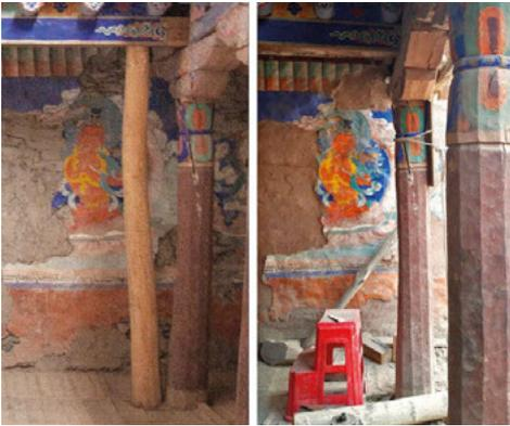
Fig. 19. Tilted structure with prop (left). The unpainted part of the beam marks the extent of the rotation of the column. The structure after it had been straightened (right).
