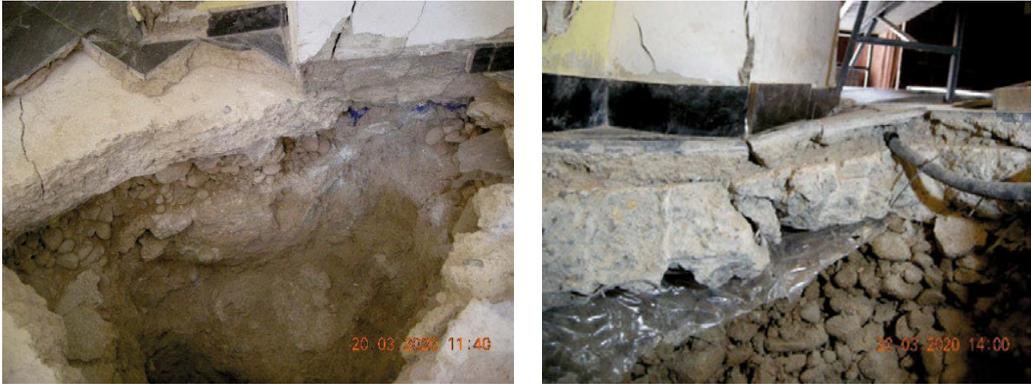
Fig. 7. Pit n°2, (interior). Next to the foundation wall of the Church. The fractured concrete floor and the foundation are recognizable. In the second photograph, detail of the deformations of the floor. Cracks are recognized in the base of the wall due to fundamentally vertical component thrusts.
