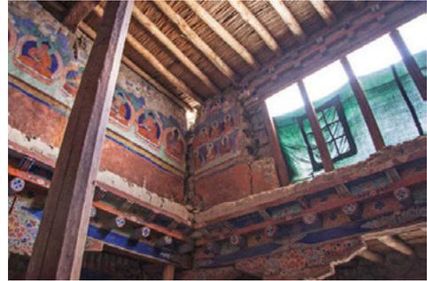
Fig. 7. The severely damaged, tilted, and detached walls on the first floor of the temple's chamber (North-west corner).
