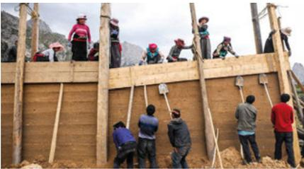
Fig.6 People were pushing up side planks of the integral formwork (Source: Shu, 2016, [https://www.poco.cn/works/detail\\_id5245000](https://www.poco.cn/works/detail_id5245000))
