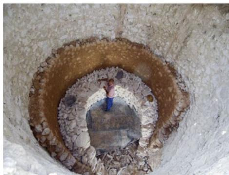
Fig. 3. Construction of the lime kiln, Morón de la Frontera, Sevilla (Juan Carlos Cazalla, 2008)
