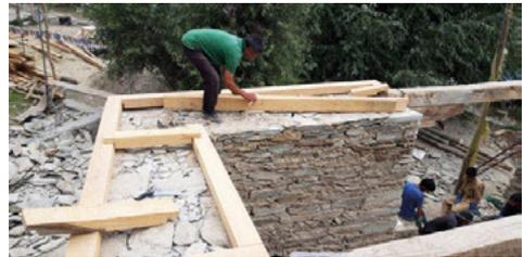
Fig. 18. Insertion of wooden tie beams (*sket shing*).
