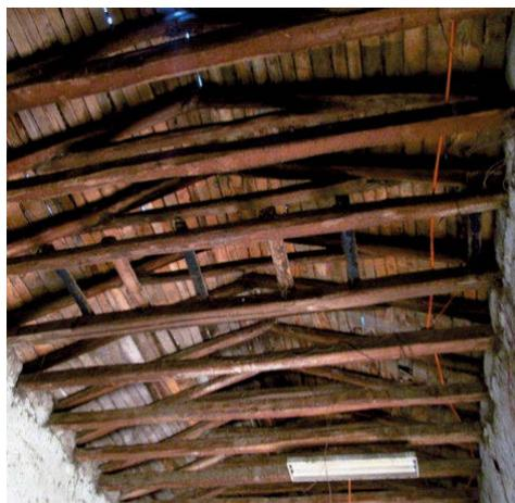
Fig. 2. Example of roof trusses on adobe walls. (Source: Contreras & Jofré, 2016)
