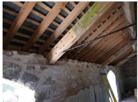
Fig. 12. Fitch plate repairs to feet of principal rafters at Great Cator (Source: White ,2021).
