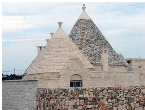
Fig. 2. Disassembly and reconstruction without preservation of original geometries (Source: Authors, 2008)
