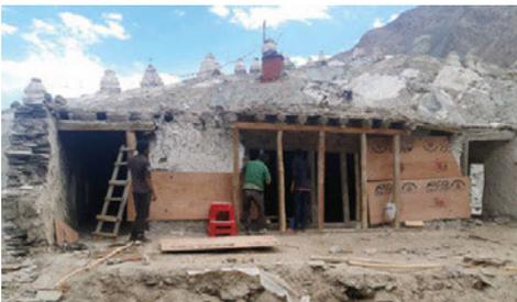
Fig. 14. Installation of plywood panels to temporarily lock the mud brick and stone walls with paintings. In the centre, a series of props are put under the cantilevered poplar beams.
