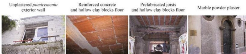
Fig. 3. Examples of inappropriate interventions on vernacular Aeolian architectures (Source: the Authors)
