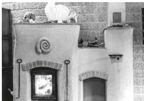
Fig. 12. Kachelofen built out of Bricks
