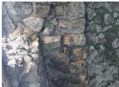
Fig. 7. Fortified house Fasano. Particular detail of the vaulting ceiling with mortar and small lava stone and arches in tuff ('spaccatelle') (Source: Ragosta, 2022).
