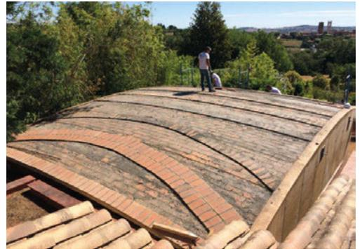
Fig. 5. Salva and Jesus Gomis working at the construction of an inclined sail-vault reinforced with ribs. This tile-vault has a 7:30 m span and a rise of 25 cm on the back and 12 cm on the front. (Source: Vitti)
