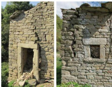
Fig. 7. Vertical bending and overturning mechanisms.
