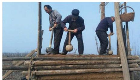
Fig.4. Rafter method used in Shanxi (Source: Zhang, 2017)
