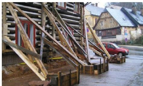
Fig. 1. Façade of the pub “Dřevěnka Inn” No. 92 (house formerly) supported by interim oblique back shores with balk and stone footing that is secured by iron anchor rods in the drilled opening, Úpice Village, Trutnov District, Hradec Králové Region © Martin Cernansky, 2008, NHI
