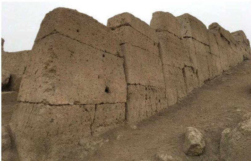
Fig. 1. A segmented wall, built by modelled earth in Tambo Inga archaeological site - Lima (Source: Torres, 2021).
