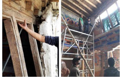
Fig. 10. Tilted wooden opening on the first floor (left); covering the paintings with a protective cloth near the wooden window (right).
