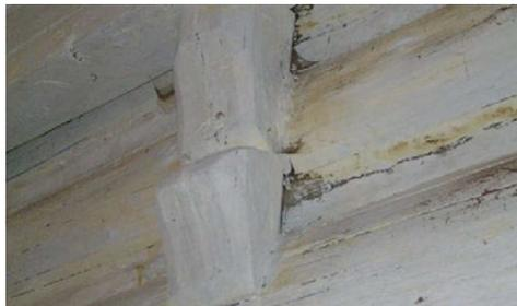
Fig. 5. House No. 53 built of logs used for walls and ceiling. Apart from this profiled bracket, there are also simple shape brackets under the supporting beam. Rtyně v Podkrkonoší Village, Trutnov District, Hradec Králové Region © Martin Cernansky, 2008, NHI
