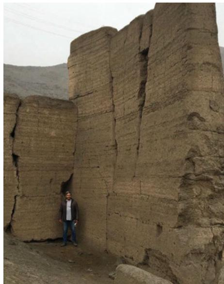
Fig. 8. Modelled earth wall, showing the layers of mud and the segmentation that allowed the displacement of the blocks. Fortress of Campoy- Lima (Source: Torres, 2021).
