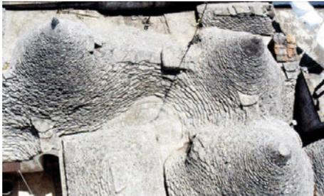
Fig. 5. Plastic solutions - without geometric regularities - resulting from empirical knowledge of rainwater runoff. (Source: Ambrosi, 1990)
