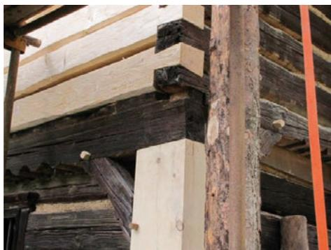
Fig. 3. Watermill No. 2 (82) and new members instead of damaged ones, the replacement requires additional supports and load securing, e. g. by carrying straps/webbing on the right, Zubrnice Rural Reservation, Ústí nad Labem District, Ústí nad Labem Region © Martin Cernansky, 2015, NHI
