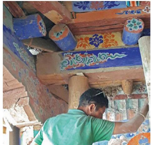
Fig. 11. One of the main beams slid 25cm outside its original position (North-eastern corner).
