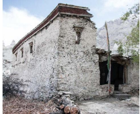
Fig. 4. Main entrance and porch. The temple started to shift from this corner at the base of the walls (North-east).
