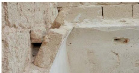
Fig. 15. 'Realina' tiled vault spring (Source: Mami, 2018)
