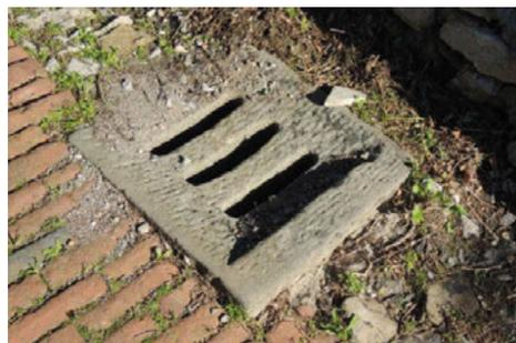
Fig.5. Sandstone storm drain (Source: Fabio Fratini).
