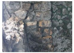
Fig. 7. Fortified house Fasano. Particular detail of the vaulting ceiling with mortar and small lava stone and arches in tuff ('spaccatelle') (Source: Ragosta, 2022).
