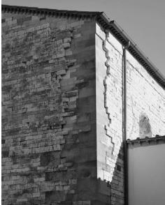
Fig. 3. damage to the wall caused by the earthquake in 1542. Church of Sant'Agata, Mugello (Source: Bordoni,
