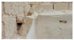
Fig. 15. 'Realina' tiled vault spring (Source: Mamì, 2018)
