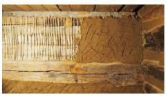
Fig. 4. House No. 14 and mud plaster application on reed mesh, the plaster is coarsened for easy topping coat adhesion as well as prevention of shrinkage cracks, Lhota Rural Reservation, Česká Lípa District, Liberec Region © Martin Cernansky, 2020, NHI
