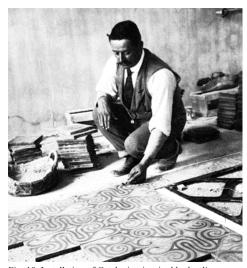
Fig. 10. Installation of Catalonian-inspired hydraulic cement mosaics or tiles. (Source: del Cueto, 2016).
