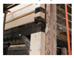
Fig. 3. Watermill No. 2 (82) and new members instead of damaged ones, the replacement requires additional supports and load securing, e. g. by carrying straps/webbing on the right, Zubrnice Rural Reservation, Ústí nad Labem District, Ústí nad Labem Region © Martin Cernansky, 2015, NHI
