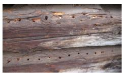
Fig. 6. Watermill No. 2 (82) and improving material properties using resin injection, Zubrnice Rural Reservation, Ústí nad Labem District, Ústí nad Labem Region © Martin Cernansky, 2015, NHI
