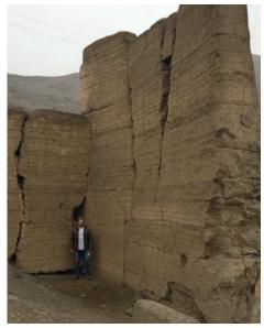
Fig. 8. Modelled earth wall, showing the layers of mud and the segmentation that allowed the displacement of the blocks. Fortress of Campoy-Lima (Source: Torres, 2021).
