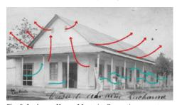
Fig. 9. Lacharme House, Monteria. Convection current ventilation, upper blinds for air renewal. Use of internal terraces to generate microclimates. (Source: Authors, 2021)
