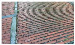
Fig.7. New, smooth bricks on which a thin biological patina is forming (Source: Fratini).
