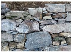
Fig. 1. An authentic stone-dry walls made using the Moltrasio limestone (Photographed by the author, January 2022)
