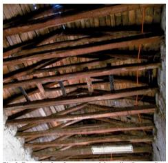
Fig. 2. Example of roof trusses on adobe walls. (Source: Contreras & Jofré, 2016)
