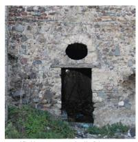
Fig. 5. Fortified house Fasano, detail of the access to ground floor: note the masonry construction 'a cantieri' and the flattening surface of the masonry section using brick elements (Source: Ragosta, 2022).
