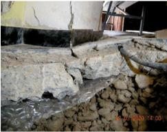
Fig. 7. Pit n°2, (interior). Next to the foundation wall of the Church. The fractured concrete floor and the foundation are recognizable. In the second photograph, detail of the deformations of the floor. Cracks are recognized in the base of the wall due to fundamentally vertical component thrusts.
