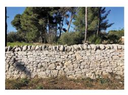
Fig. 5. Detail of a dry stone wall (Source: Farina, 2021).
