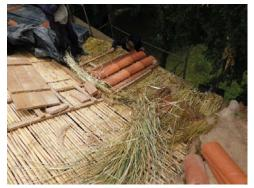
Fig. 8. Eaves with plant fibre fabrics in Casa del Marques ©
