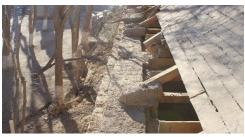
Fig. 5. Detail of the reinforced concrete beam incorporated into the adobe walls in Casa del Marques @ Authors
