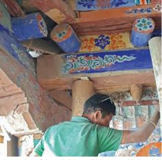
Fig. 11. One of the main beams slid 25cm outside its original position (North-eastern corner).
