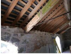
Fig. 12. Flitch plate repairs to feet of principal rafters at Great Cator (Source: White ,2021).
