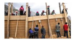
Fig.6 People were pushing up side planks of the integral formwork (Source: Shu, 2016. https://www.poco.cn/works/detail\_id5245000)
