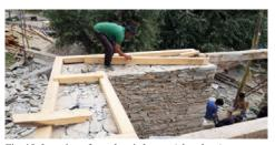
Fig. 18. Insertion of wooden tie beams (sket shing).
