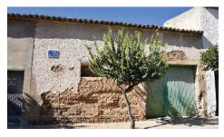
Fig. 6. Vernacular adobe building with visible erosion.
