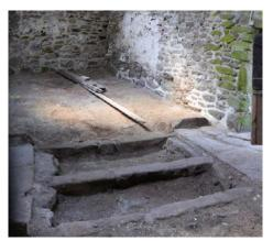
Fig. 9. Sleeper walls of former suspended threshing floor (Source: White, 2021).
