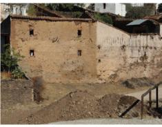
Fig. 2. Housing built with raw earth. Hinojales, Huelva.(Aniceto Delgado Méndez, 2019)
