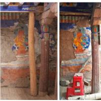
Fig. 19. Tilted structure with prop (left). The unpainted part of the beam marks the extent of the rotation of the column. The structure after it had been straightened (right).
