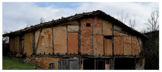
Fig. 2. Building in Villanueva de Tobera (Burgos), showing material lesions (damp stains, erosion, loss of volumetry, rot, replacement of infill, elimination of structural elements) and structural lesions (excessive buckling of timber, lack of bonding and fissuring of the infill) (Source: Hueto-Escobar, 2022).
