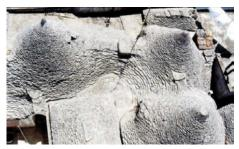
Fig. 5. Plastic solutions - without geometric regularities resulting from empirical knowledge of rainwater runoff. (Source: Ambrosi, 1990)
