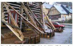
Fig. 1. Façade of the pub "Dřevěnka Inn" No. 92 (house formerly) supported by interim oblique back shores with balk and stone footing that is secured by iron anchor rods in the drilled opening, Úpice Village, Trutnov District, Hradec Králové Region © Martin Cernansky, 2008, NHI
