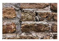
Fig. 4. Detail of medieval brickwork with well-polished limeand-sand repointed joints (on the right) and a modern addition with a Portland cement mortar joint (left) highlighting the loss of traditional building skills (Source: Squassina, 2021)
