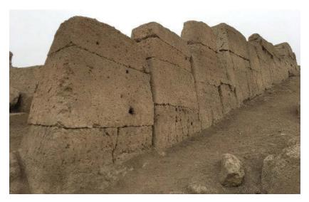
Fig. 1. A segmented wall, built by modelled earth in Tambo Inga archaeological site - Lima (Source: Torres, 2021).
