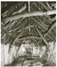
Fig. 3. Cruck framed roofs ensured the stability of roofs, Dumfriesshire - Scotland (Source: Walker, McGregor, Conservation of Vernacular Buildings).
