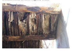
Fig. 9. Fortified house Casillo, Wooden ceiling with chestnut beams and second-arybeams ('chiancarelle') and flooring stratigraphy (Source: Ragosta, 2022).
