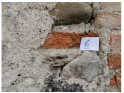
Fig. 11. Analysed ancient brick (Source: Fratini).
