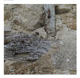
Fig. 5. Detail of the half-timbered wall with stone in Viveiro (2021), (Source: AFP).
