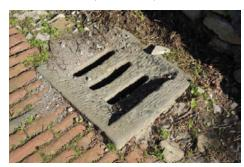
Fig.5. Sandstone storm drain (Source: Fabio Fratini).
