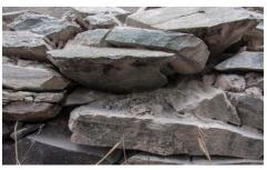
Fig. 5. Bulging plinth with eroded mud mortar (North-east).
