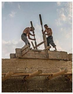
Fig.12 The formwork used in Tulou (Source: Chen, 2016, www.163.com/dy/article/E9GLU3K10521AJ1J.html)
