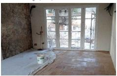
Fig. 10. Clay tiles already placed in living room, waiting for minimum 25 days complete drying (Source: Li Puma, 2021)
