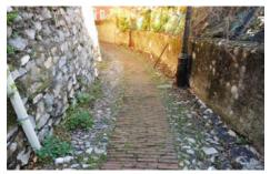
Fig.3. Genoa, crêuza with lateral cobble-stones and central brick strip (Source: Fratini)
