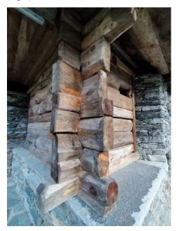
Fig. 4. Detail of the Blockbau technique at the House 2: half-log walls joined at the corners (Source: Di Paola).
