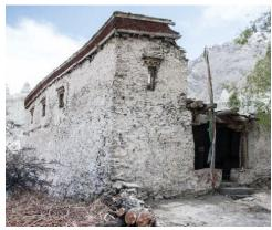
Fig. 4. Main entrance and porch. The temple started to shift from this corner at the base of the walls (North-east).
