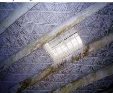
Fig. 4. Traditional Ceiling, ith palm trunks, palm stems and a shaft.
