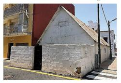
Fig. 7. Isolated Valencian barraca, in a distric of Valencia. This traditional local architecture is made of adobes, and it was once primarily spread around the city's territory. Today only a few examples have endured, and most of them are surrounded by the presence of modern buildings which have no connection with the traditional architecture and urban morphology (Source: Caruso, 2018).
