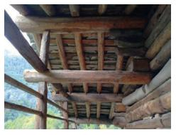
Fig. 5. Detail of the structure of the roof built with three frames, carrying stone labs (Source: Di Paola).
