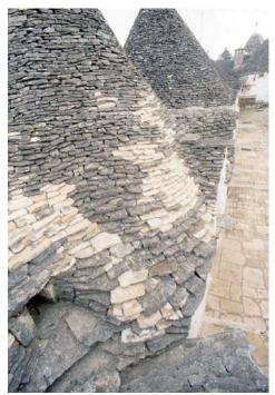
Fig.7. Conservative replacement operation respecting geometric-formal solutions. (Source: Ambrosi, 1990)
