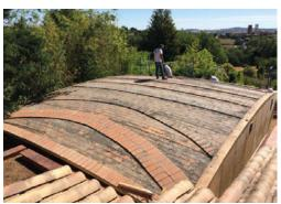
Fig. 5. Salva and Jesus Gomis working at the construction of an inclined sail-vault reinforced with ribs. This tile-vault has a 7:30 m span end a rise of 25 cm on the back and 12 cm on the front. (Source: Vitti)
