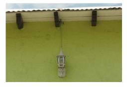
Fig. 1. Replacement of curved clay tile roof with galvanized sheets. (Parra Zebadúa., 2021)
