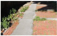
Fig.6 The installation of water systems has damaged the paving (Source: Fratini).
