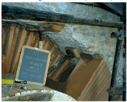
Fig. 1. Reconstruction of a Roman arch with bipedales at Domus Tiberiana, Rome. (Source: Vitti)
