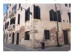
Fig. 5. New thick plasters cannot withstand the effect of rising damp for long in Venice: the above example is less than a decade old (Source: Squassina, 2021)
