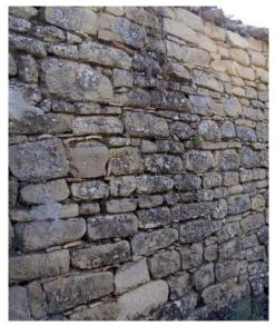
Fig. 4. Detail of a wall in Porcuna without mortar (a hueso construction). (Source: Belmondo, Millán, 2022).
