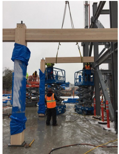
Figure 5,6. Carbon12 Detail, Beam - Steel Core Connection with adjusted glulams. Source: (Kaiser+Path n.d.)
