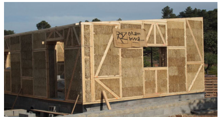
Figure 1. Construction process using rice straw panels.
